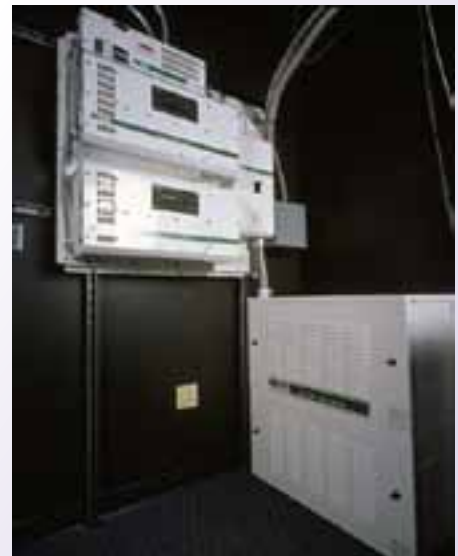
Inverters and battery storage for photovoltaic system
