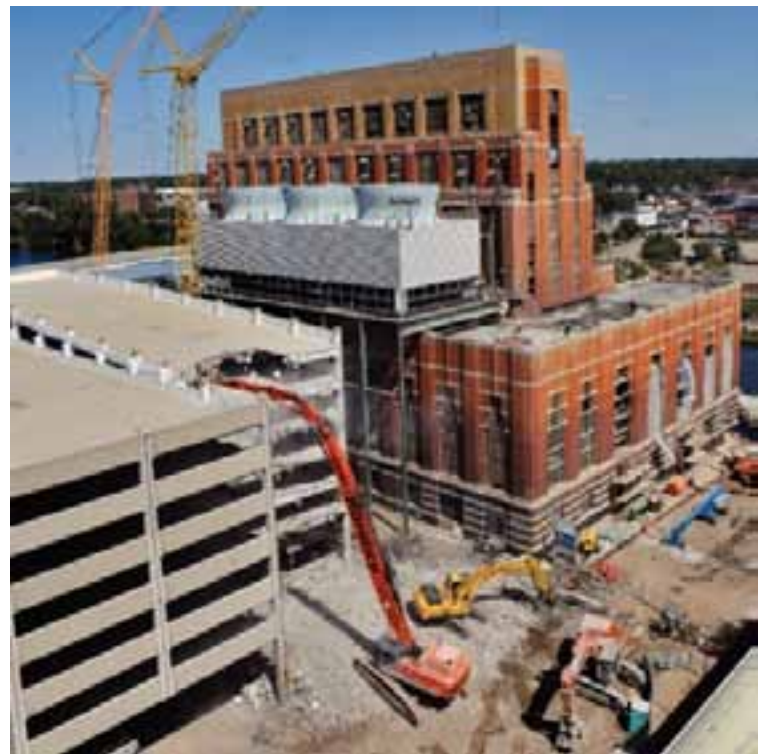
2008 – city parking ramp and chiller cooling towers under demolition.
